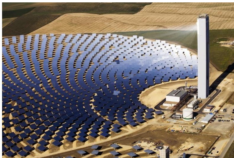
Figure 3: Solar Concentrator Thermal Power Plant [7]
